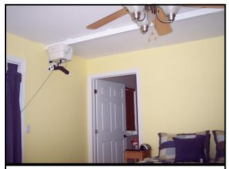
Notice the visible track? Try having a recessed ceiling track lift installed instead!
