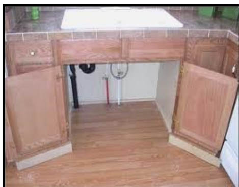
Cabinet doors revealing open space under sink
